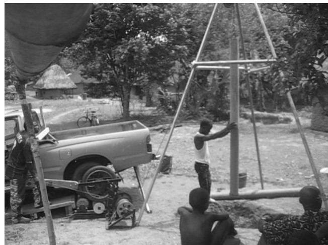
Figure 2. Drilling well in Sierra Leone
