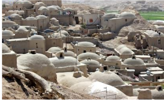
Figure 14. Employing cooling effect of shadow by dome shape roofs, Seestan Masooleh, Iran
